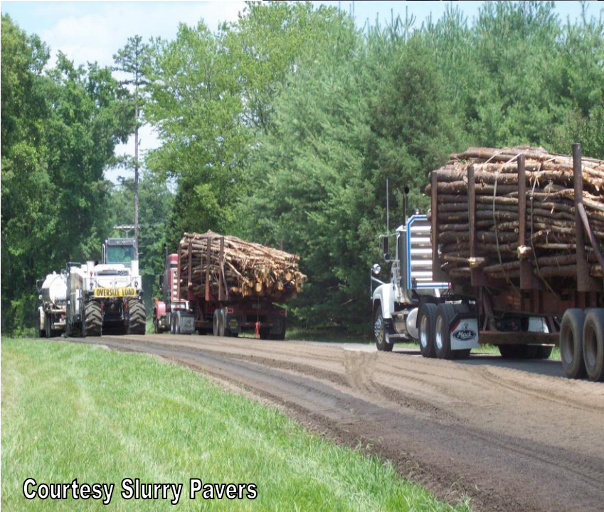
Courtesy Slurry Pavers
