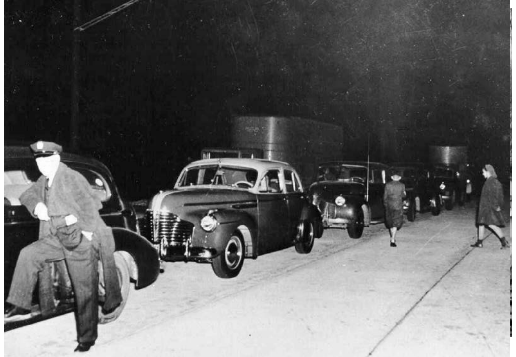
Rows of cars line up at “ticket offices” (tollbooths) to be first on the heralded highway.
