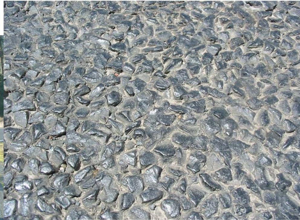
95% of all sealed roads in New Zealand are chipseal over unbound granular pavements
