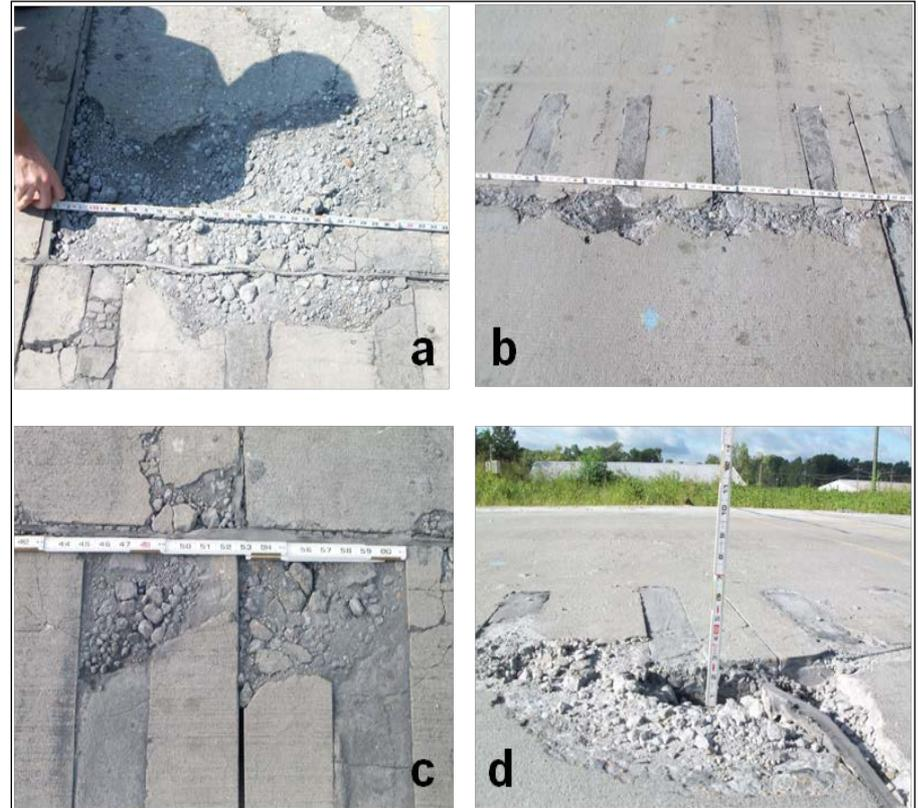
Typical Failures: Panel 1 N joint, (b) Panel 2 S joint, (c) Panels 2 and 3 N joints, (d) Panels 6 and 7 S joints
