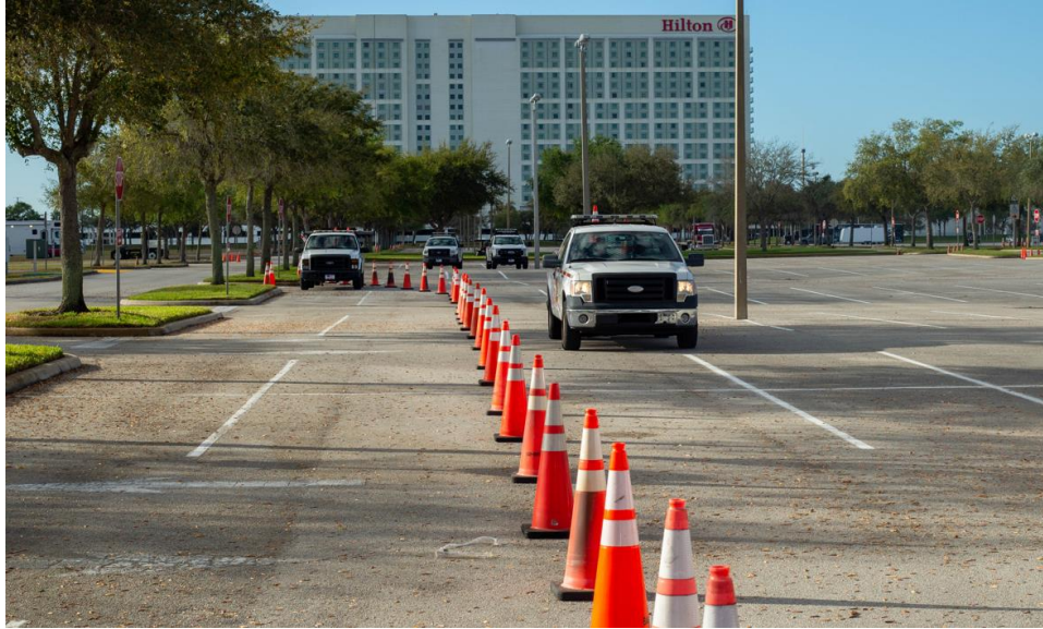
Figure 4. Photo. Work zone setup as part of the closed-course testing at the TMC Annual Meeting.
