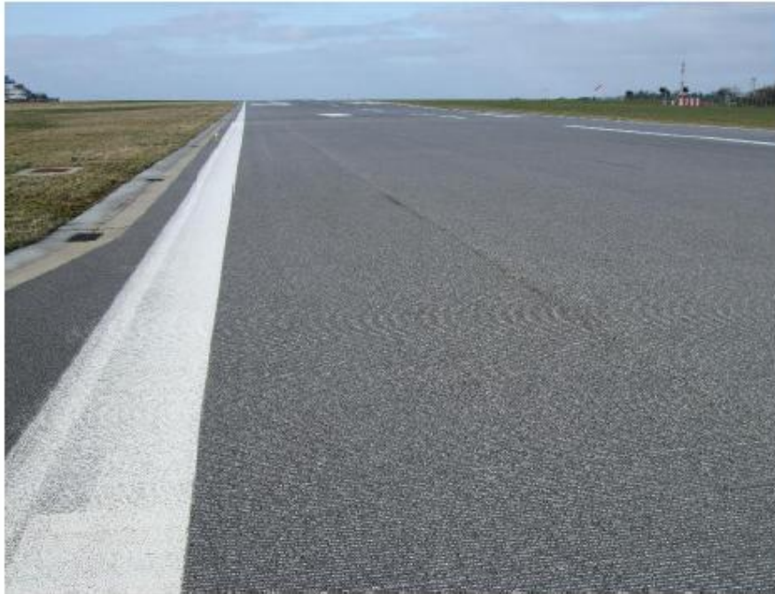
(a) Surface area generally in good condition
