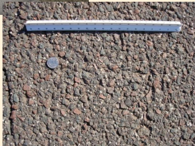
Shotblasting/Abrading
