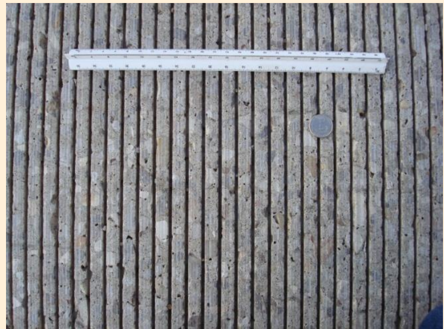
Grooving “Next Generation Diamond Grinding”
