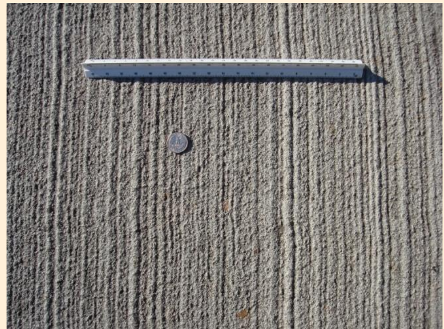
Ultrathin Cementitious Overlay
