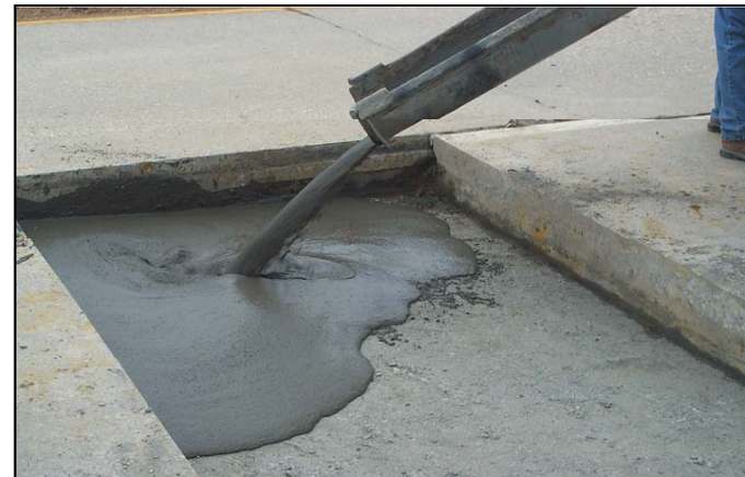
Flowable Fill Installation Detail
