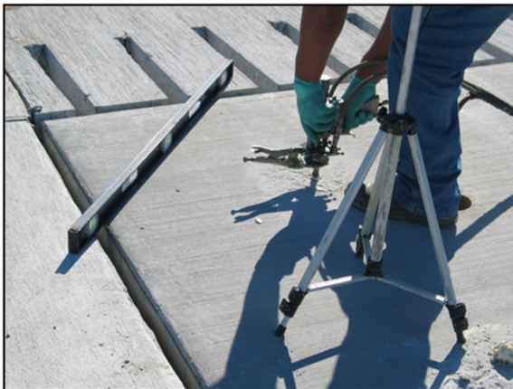
HDP Foam Injection
