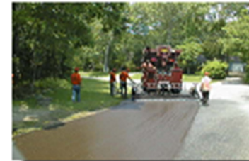
Application of skid-resistive pavement surface in curve.
