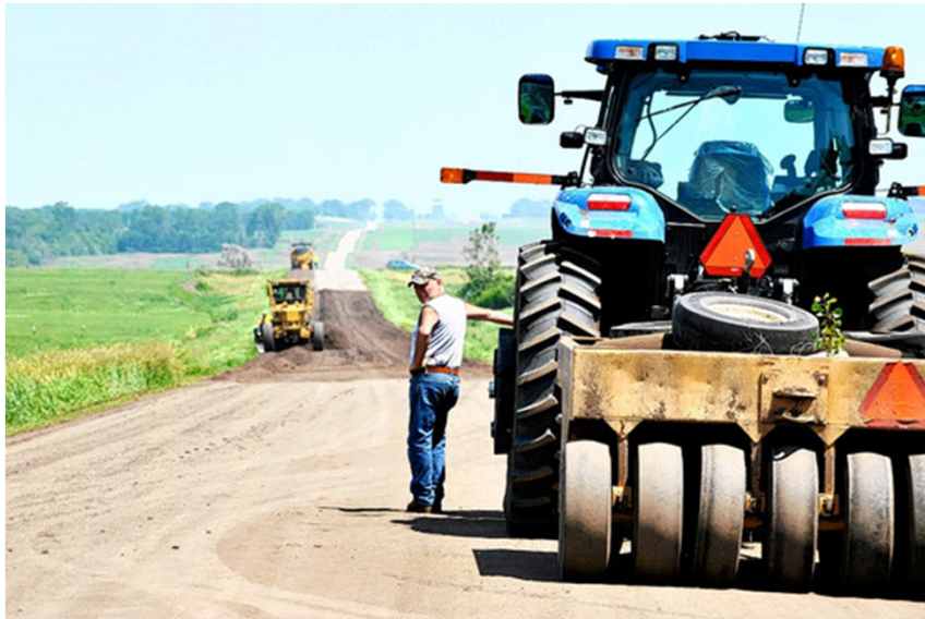
Road crew in Jamestown, N.D.; turning asphalt roads into gravel ones...
