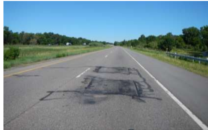
Overview of one of the sections, Source: FHWA
