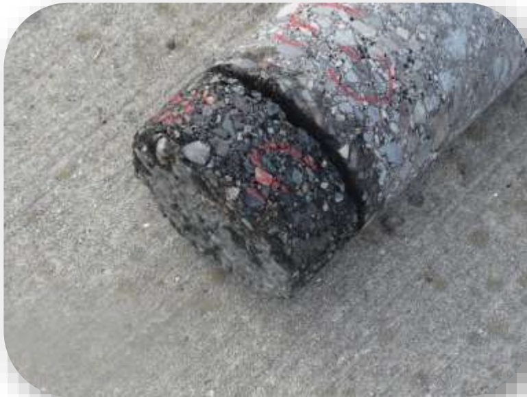
Core 3 (Slight HMA Stripping)
