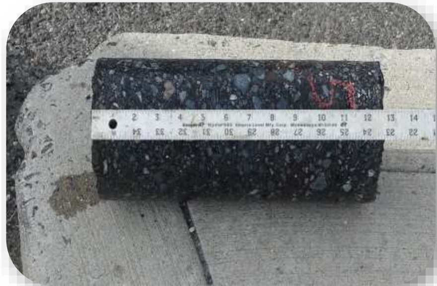
Core 5 (No HMA Stripping)
