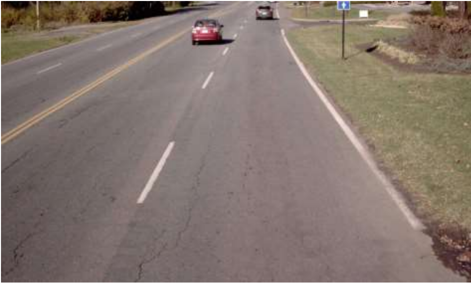
Significant visible cracking
