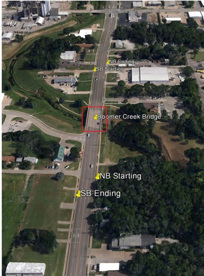
(a) Bridge Location
