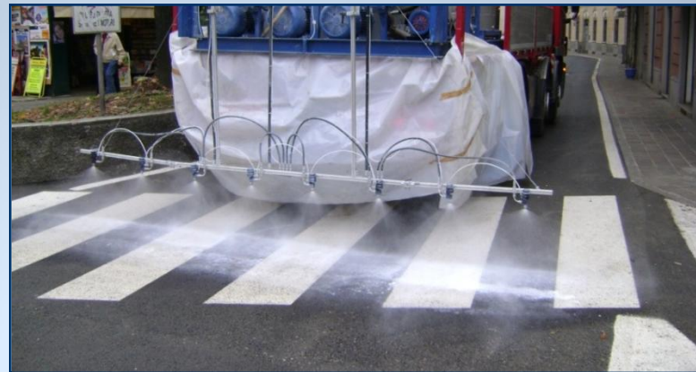
Bituminous pavement sprayed with photocatalytic pollutants/emulsions
