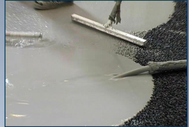
Photocatalytic pavements combining asphalt and cement mortars
