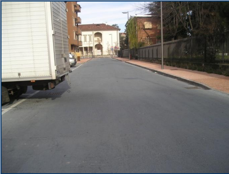
BLUE PHOTOCATALYTIC PAVEMENT Cinisello Balsamo (Milan)
